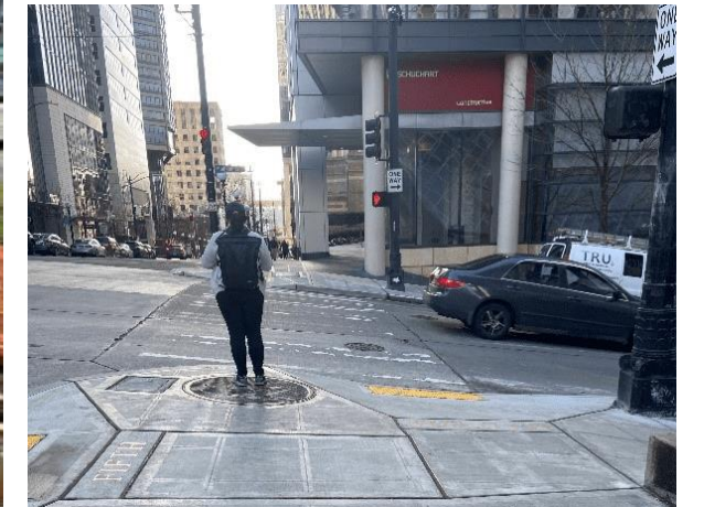
Rebuilt sidewalks and ADA-accessible ramps; shown here are new ADA curb ramps at 5th Ave and Madison St as part of RapidRide G Line project.
